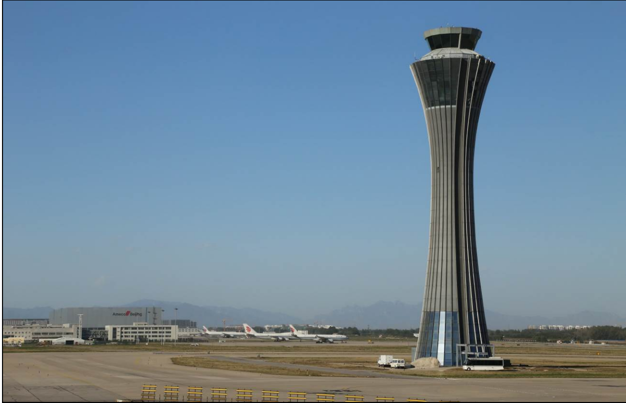
The Air Traffic Control Tower at Beijing Capital International Airport, China
